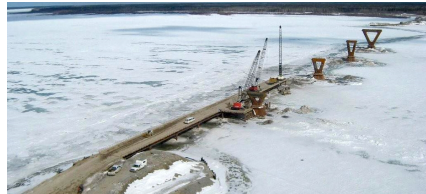
Deh Cho Bridge Construction, April 24, 2009
