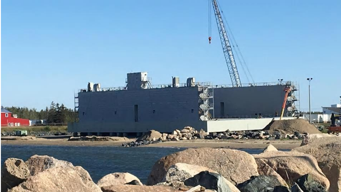
Exhibit 4.9 - Construction of the dry-dock
