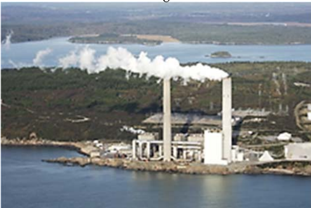
Coleson Cove Generating Station
