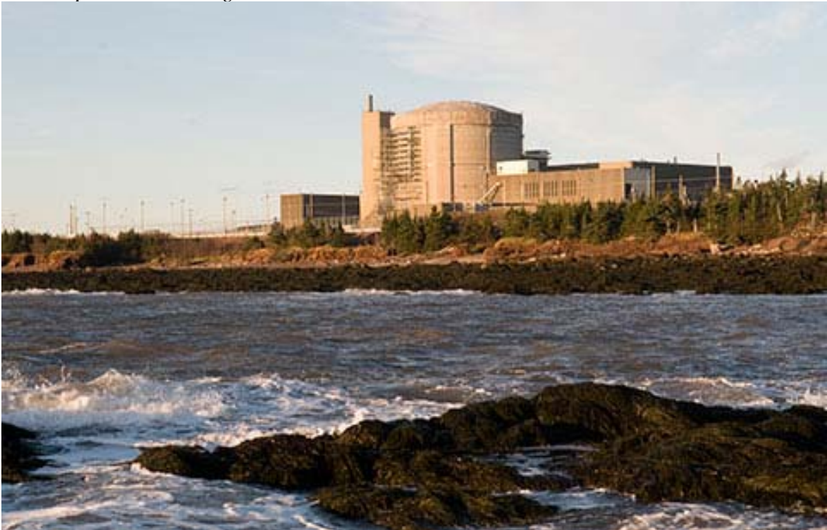
Point Lepreau Generating Station
