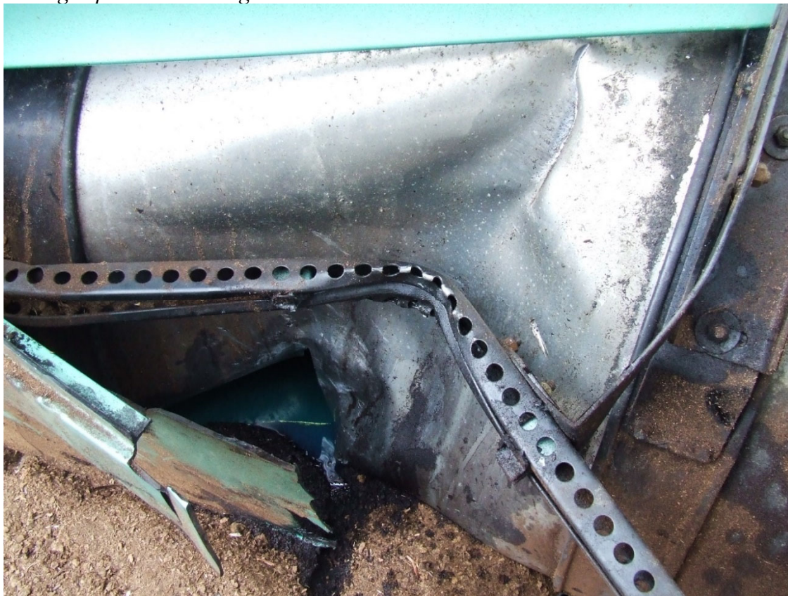
Damaged petroleum storage tank and leak
