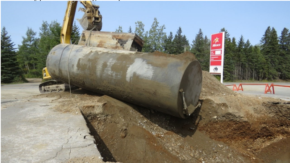
Removal of petroleum storage tank parts
