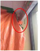
Construction areas not properly sealed at ceiling or floor
