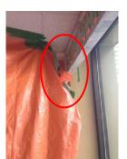
Construction areas not properly sealed at ceiling or floor
