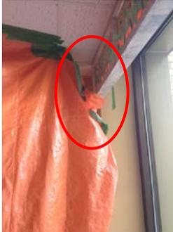
× Construction areas not properly sealed at ceiling or floor
